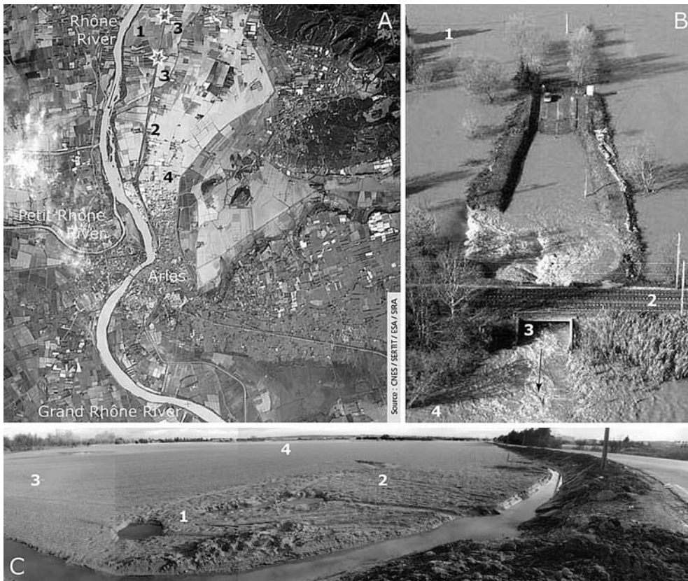
FIG. 2 - Flooded area during December 2003 flood event, on left bank of the Rhône River between Beaucaire-Tarascon and Arles. A: General view of flooded area in December 2003. 1: ségonnal ; 2: dyke (RFF railway embankment) for flood-plain protection; 3: tunnels under railway track (Rhône River floodwaters rushed through the tunnels); 4: inundated flood plain. B: Tunnel under the RFF railway track in the site of «Mas Tessier» upstream of Arles (03/12/03; photo in Degoutte & Sarralde, 2008). 1: ségonnal ; 3: tunnels built under the railway track (2) allowing Rhône River floodwaters to rush through tunnels); 4: inundated flood plain. C: Flooded area outside dyke at «La Citerne» site, upstream of Arles. After flooding of tunnel crossing the dyke (RFF railway embankment), the floodwaters that were guided by the road (to the right) invaded the flood plain. 1: scour depressions (length: 1.2 m; width: 0.8 m; depth: 0.5 m); 2: stripped zone and micro-channel cutting into surface; 3: accumulation of silts with very fine sands; 4: proximal flood basin. Photo: G. Arnaud-Fassetta (03/12/22).
