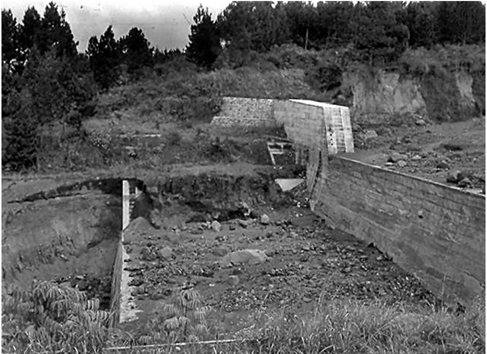
FIG. 4 - Automated warning system at a lahar check dam on the SW slopes of the Merapi volcano, Central Java, Indonesia. The arrow points to the fastening of three thin horizontal steel cables that stretch across the check dam. Note the rise of the valley floor caused by the structure.
