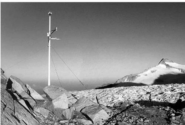
FIG. 3 - The Passo della Lobbia Alta (3020 m a.s.l.) meteorological station. Wind speed and direction, air temperature and humidity, incoming and reflected global radiation and net radiation are measured. The photograph was taken on the 17 th of August 2001, eight days after the installation. On the right: Crozzon di Lares peak (3354 m a.s.l.).
