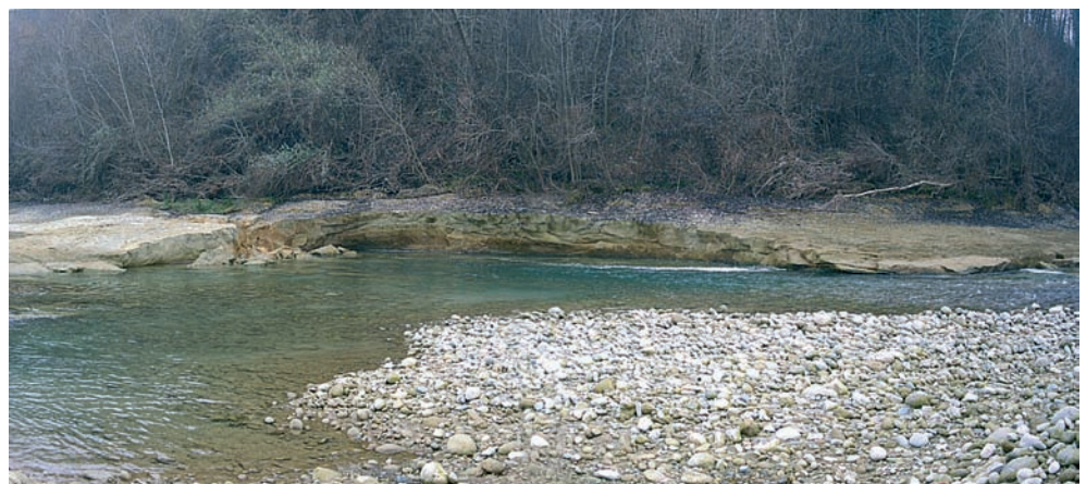
FIG. 6 - The Orco River 1.5 km upstream of the Feletto bridge in January 2007 (downstream to the left). Since the beginning of the 1980s the vertical erosion has incised the lacustrine deposits previously buried by fluvial deposits.
