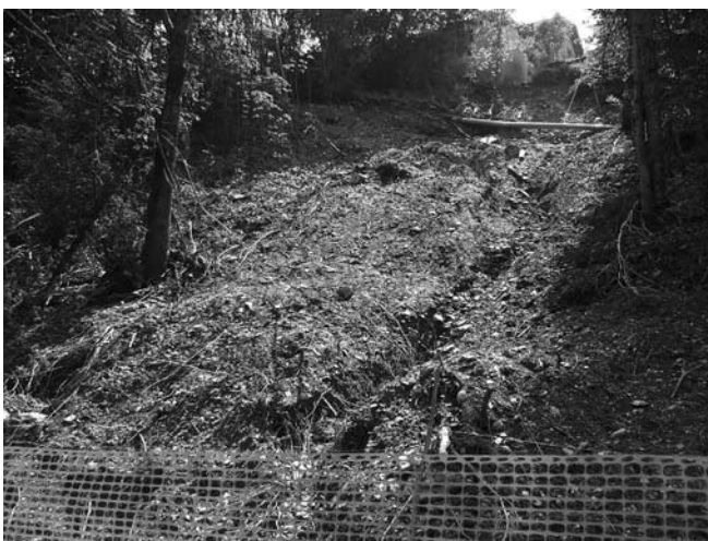
FIG. 9 - Rotational landslide near Campo la Salza. Note the sewer pipe exposed by the landslide.
