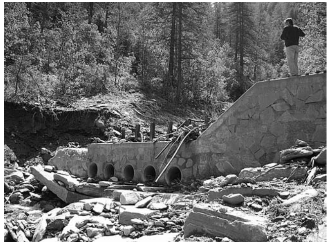
FIG. 8 - Apex of the alluvial fan of the Rio Iclo. Deep erosion; the right shoulder of the weir has been completely washed away. Just downstream from the weir, to the left, note the differences in rock size: scattered large rock masses and a fine matrix composed of sand and gravel.
