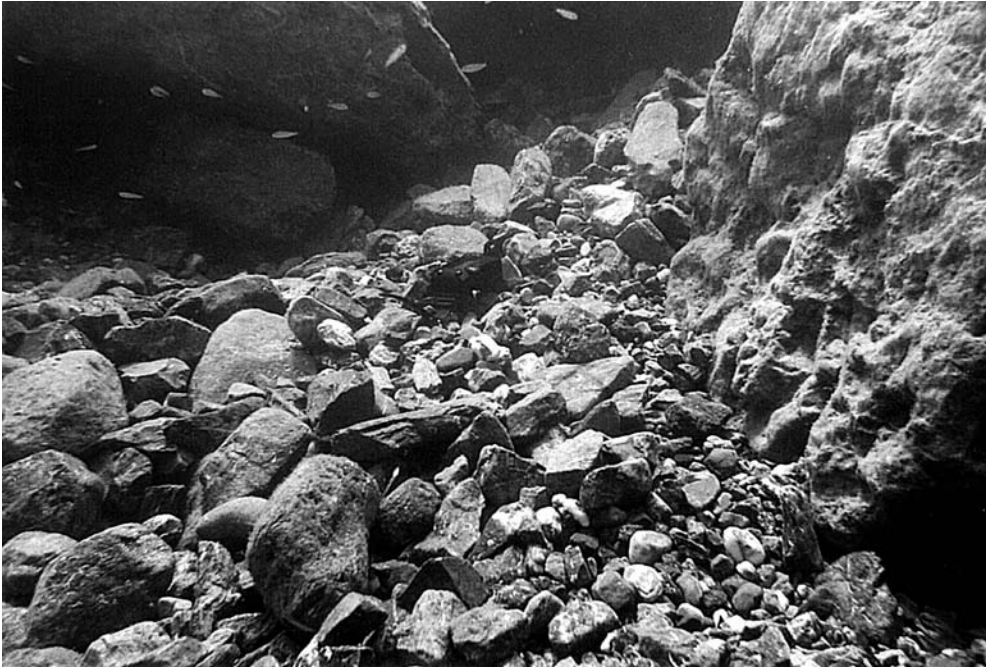
FIG. 8 - Detail of the seafloor close to a breakwater.
