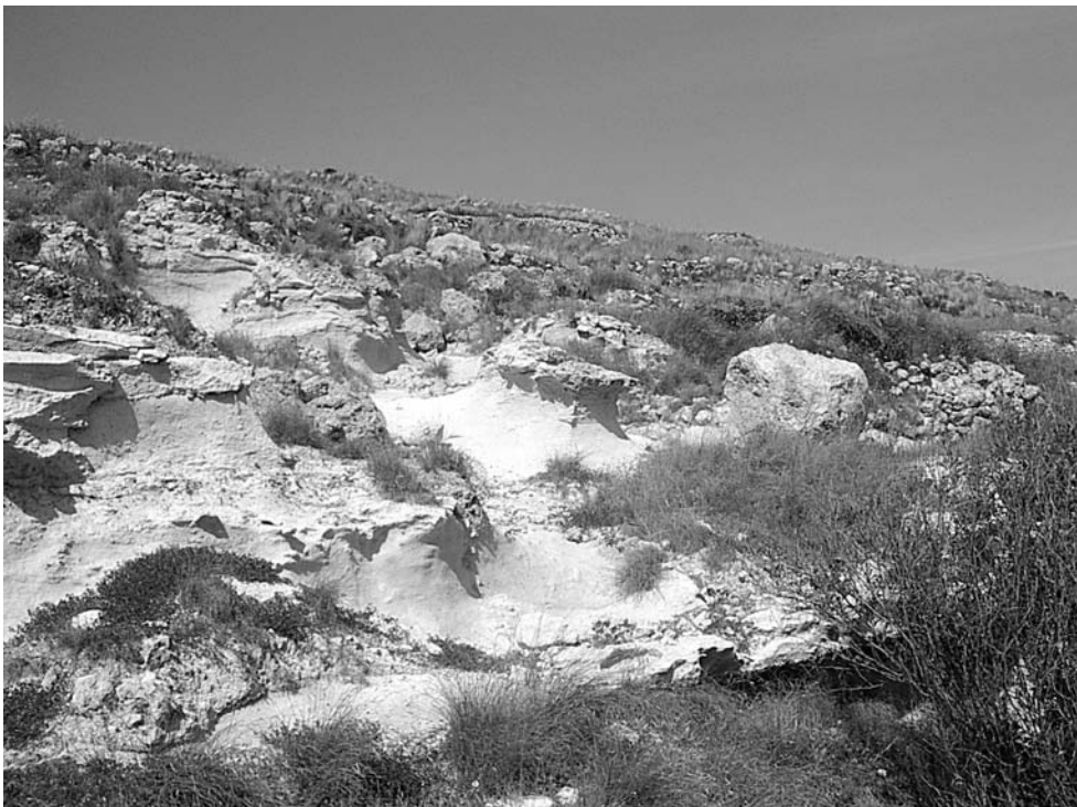
FIG. 2 - Erosion on abandoned field terraces, Gnejna Valley, Malta. Bedrock is Middle Globigerina Limestone, slope angle ranges from 10 to 15 degrees. Photo B. Cyffka, September 2004.
