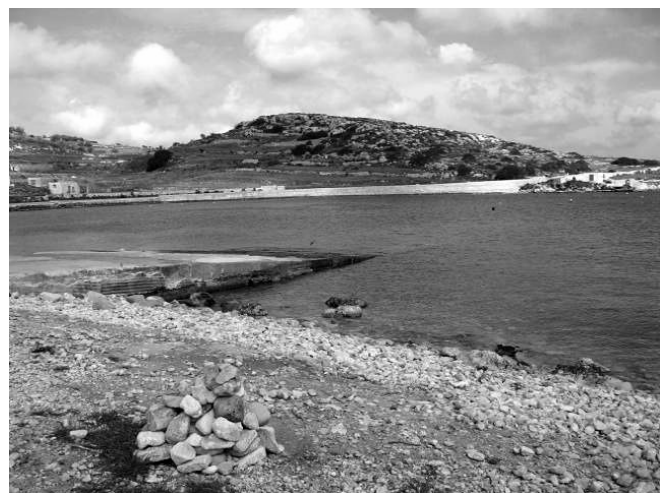
FIG. 6 - Coastal structures at Mistra Bay.
