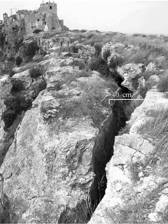
FIG. 8 - Tensile failure within the upper rigid formation at San Nicola.
