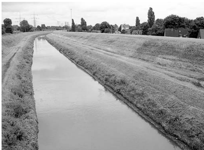
FIG. 6 - The channelized and diked river Emscher in the city of Herne (photo by J. Herget).
