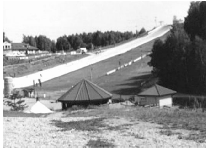
FIG. 3 - Artificial ski track built of waste dolomite from a quarry in Bytom (photo by J. Pelka-Gosciniak).
