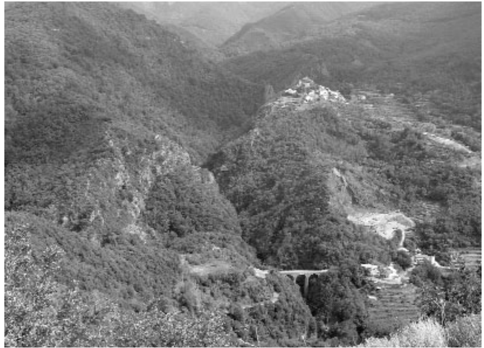
FIG. 8 - Ponte di Lagoscuro gorge: pillow lavas in the Graveglia valley (bridge in the foreground), extracted in the Molana quarry (on the right); the cherts outcrop in the Novelli stream climbs up to Nascio hamlet. At left of Nascio hamlet is the Novelli gorge, carved in the cherts and basalts, at the confluence of Graveglia stream.
