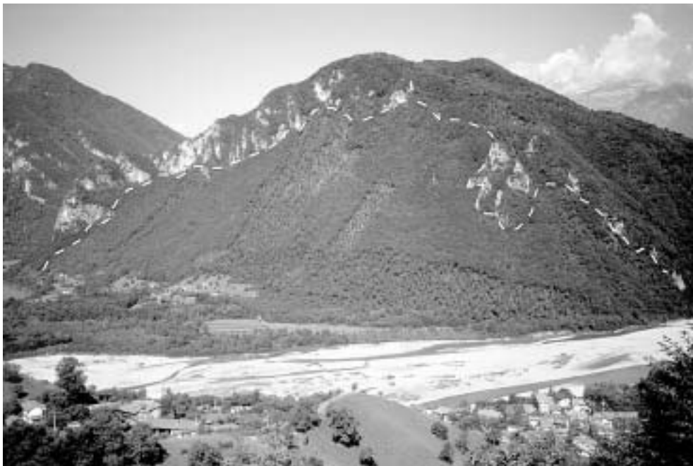
FIG. 7 - The Marziai landslide (the dashed line shows the scar); in the foreground the Marziai village and the Piave River.
