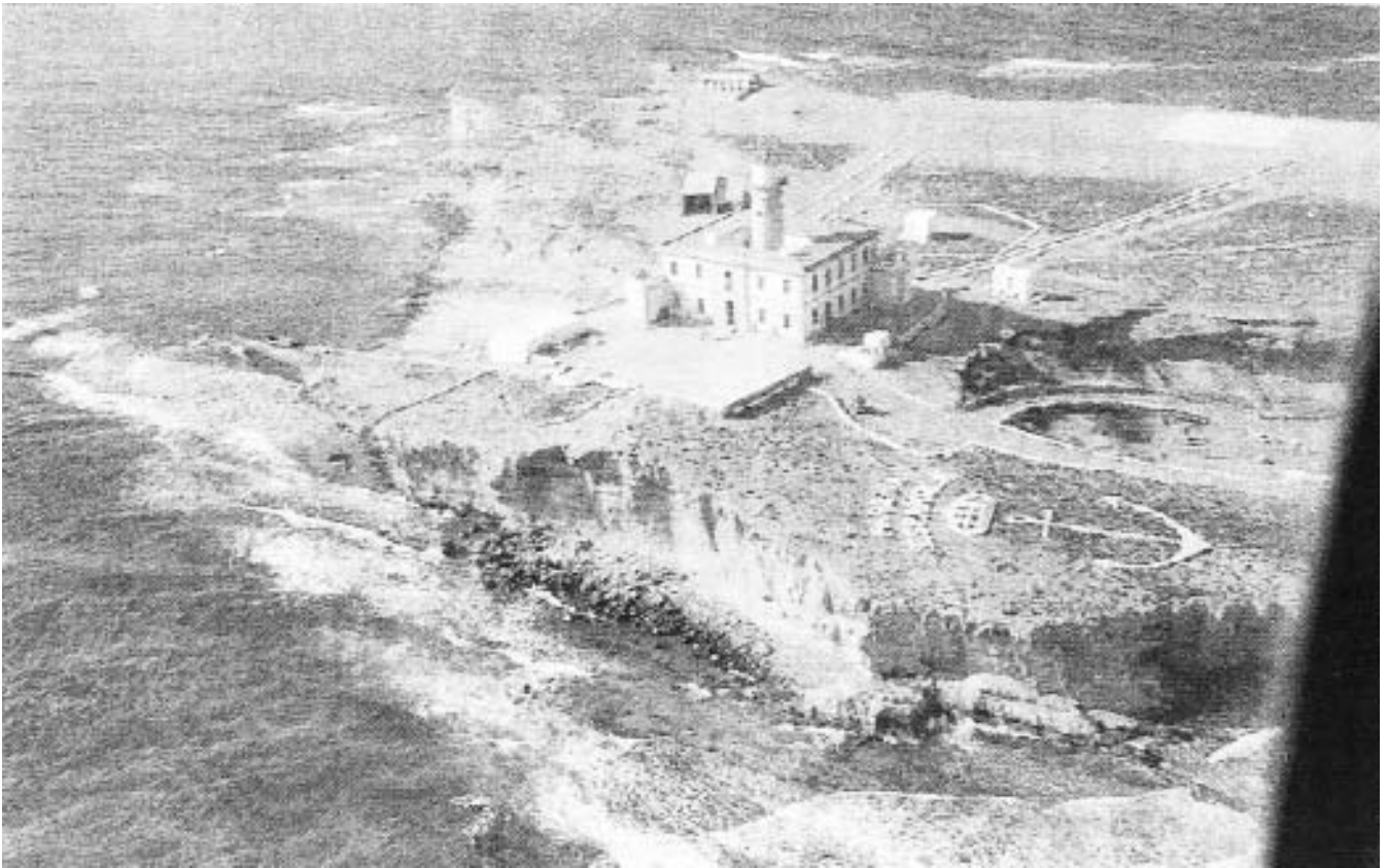
FIG. 8 - Oblique aerial view of the lighthouse (1978).
