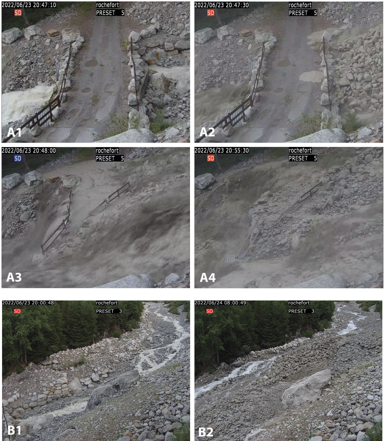
FIG. 6 - Sequence of images of the Rochefort bridge that crosses the Montitaz Stream. A1 to A4 are images of the camera surveying the bridge when the debris flow impacted the bridge h 20:47-h 20:55. B1 and B2 are images of the camera surveying the Montitaz Stream just above the bridge at h 20:00 before and at h 08:00 the morning after the event. A significant deposition of debris is evident.
