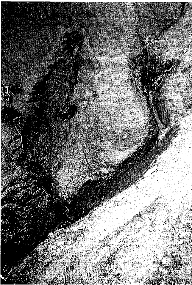
FIG. 4 - Rill cutting gully side of Grosse Pierre (anticlinal depression of Sederon). Roof of pipes have broken down and «gorges» are cutted as far as fresh marls. Instability of sides of these gorges is identified by cracks. (Site D).
