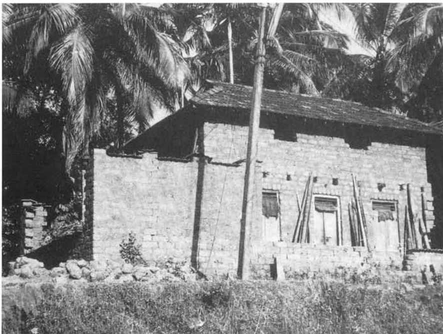
FIG. 5 - A traditional two-storey house under construction in 1982. Chellur, Kerala.
