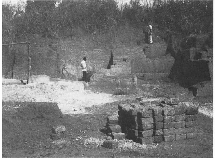
FIG. 4 - Excavation of laterite for a house, Chellur, Kerala. Part of the house is excavated, and the excavated blocks will be used for building walls. A well has been sunk on the left, and pallid zone material has been brought up.
