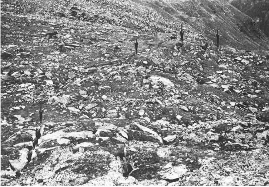
FIG. 7 - Open tension cracks striking in various directions, which dissect the topography on the western slope of Valle del Pasquale. They are indicated with black arrows.
